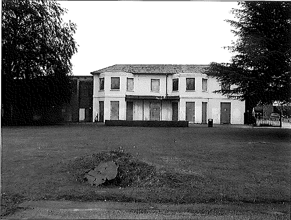
Photo showing the south east elevation of Brightwell House and the adjoining Redgrave Theatre.
